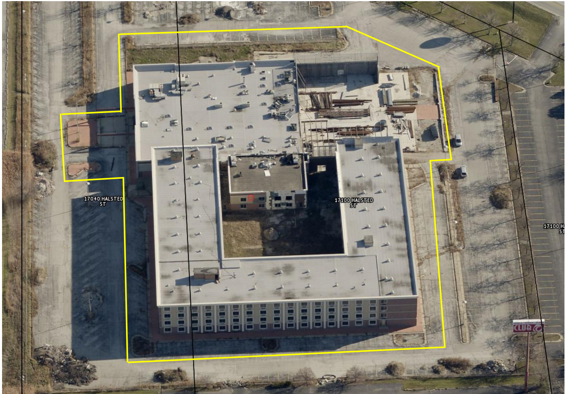
17040 S Halsted, Harvey Demo – Work Area (West Façade View)
